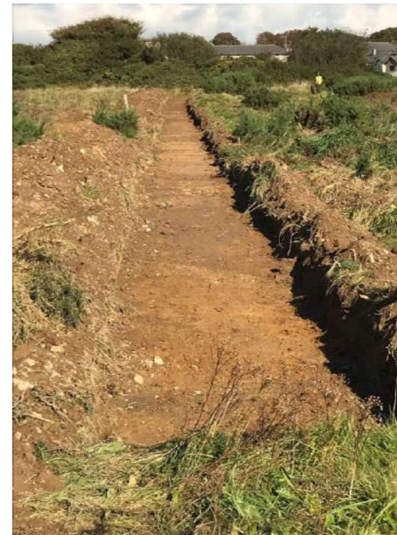
Plate 1 Trench 7, facing north
