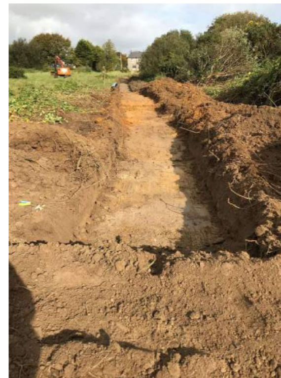
Plate 3 Trench 17, facing north
